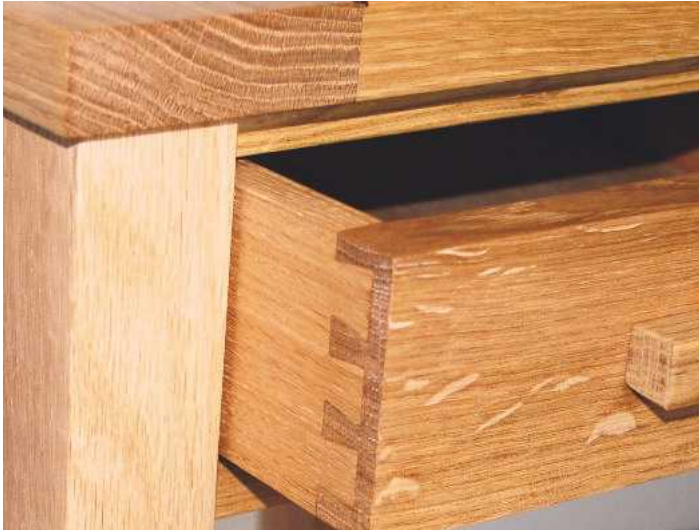
▲ Pic.9 The lapped dovetails keep the lines of the drawer front clean...
